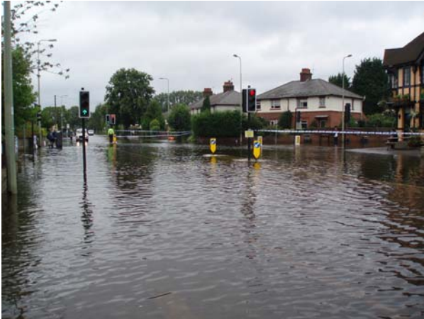
Flooding in Oxford in 2007
