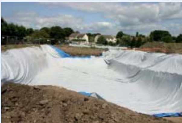
Stage 3: Put root barrier membrane in place, allowing enough material along the edges to eventually provide a seal.
