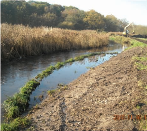
5. Low level berm installed to diversify flows in existing river channel
